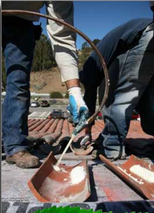
Polyset® is the professional roofer's complete solution for concrete or clay roof tile attachment. Polyset® is a patented polyurethane adhesive that adheres each individual tile in place. It can be used without mechanical fasteners so it won't puncture the waterproofing membrane or roof deck. Polyset has superior holding power compared to nails, screws, mortar and wire tie systems.
