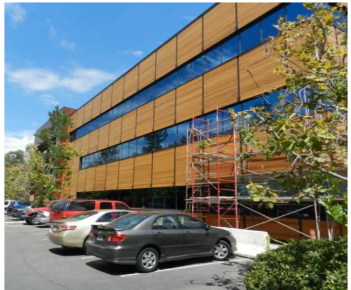
Climate-Shield rain screen system using reclaimed 1x6 redwood siding
