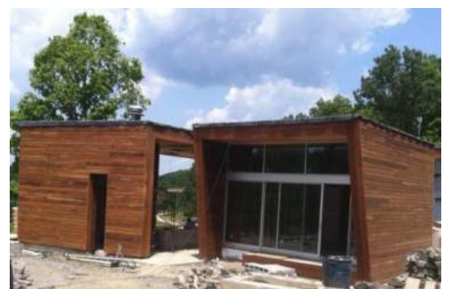
1 x 6 lpe rain screen cladding with mitered outside corners
