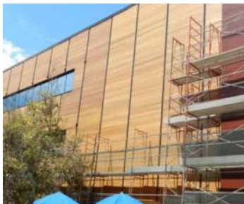
Climate-Shield rain screen system using reclaimed 1x6 redwood siding
