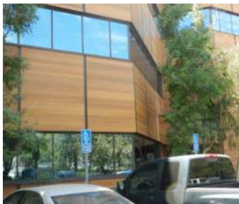
Climate-Shield rain screen system using reclaimed 1x6 redwood siding
