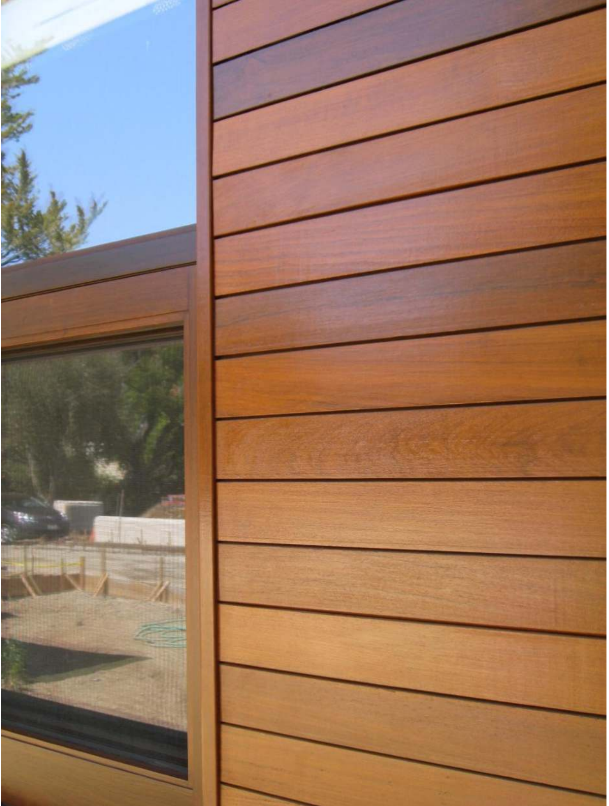
Window trim detail using 1x6 Ipe cladding in rain screen design Weeksville Heritage Center, Brooklyn New York
