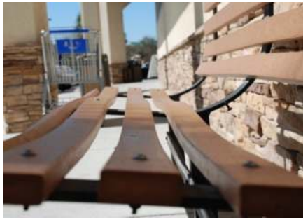
Plastic decking "sagging"
