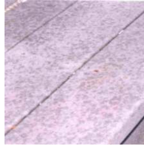
"Composite decking" exhibiting fading and permeation of mold and mildew
