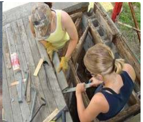
Replacement of dryrot porch flooring
