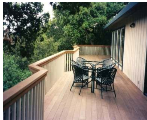
Hardwood deck with traditional railings
