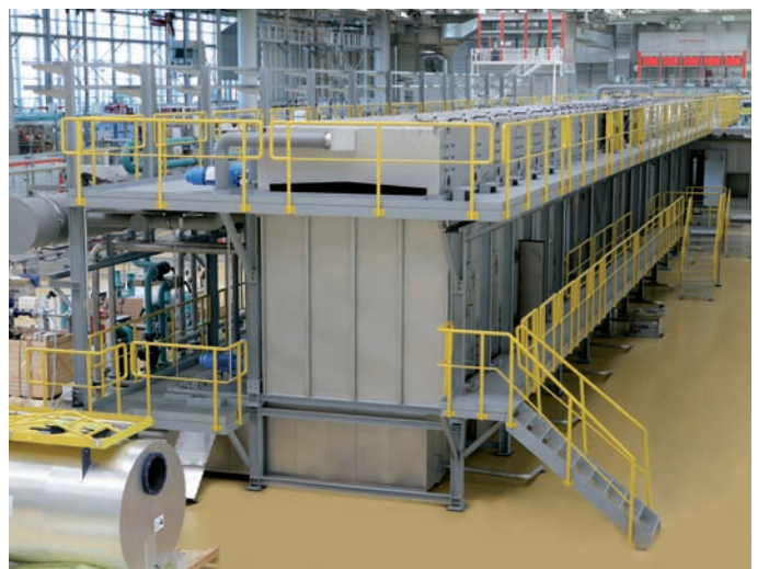
Pretreatment for paint lines
