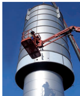
Assemblage of a loop reactor.
