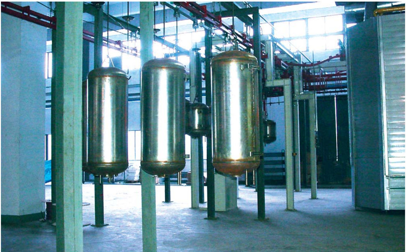
Fig. 3: Power&Free transport of the coated boilers to enamel firing at approx. 850 °C
