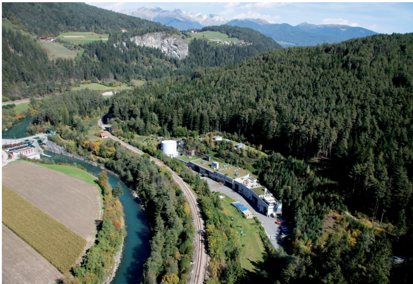
Picture 7: The public wastewater treatment plant of Central Puster Valley is hidden inside a mountain. Only administration, sewage sludge drying and the Pyrobustor® plant for thermal sewage sludge utilization are located above the ground.
