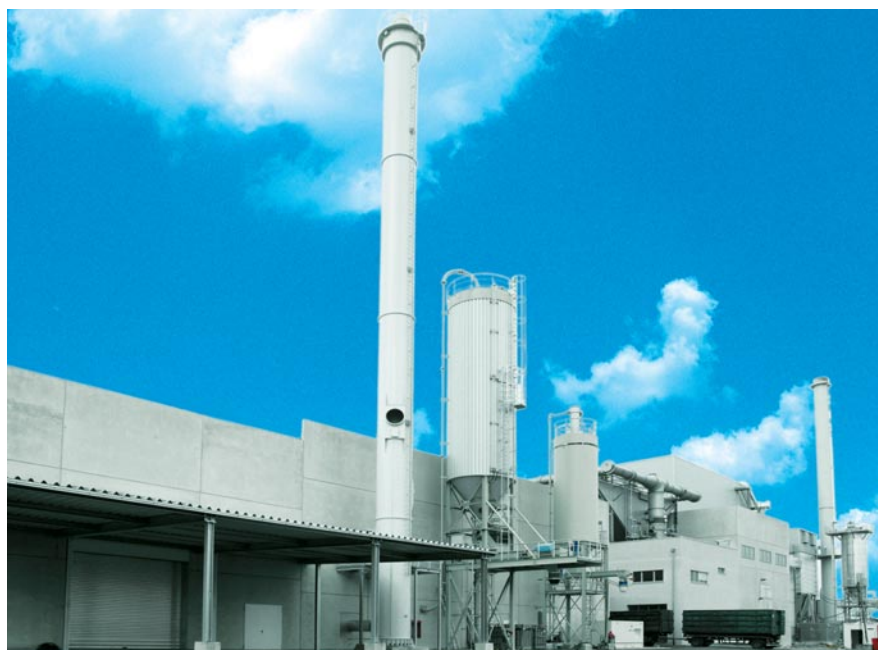
Picture 3: The hitherto unique combination of a biomass-fueled power plant and Pyrobustor® for the thermal utilization of sewage sludge, known as the "Crailsheimer Model".
