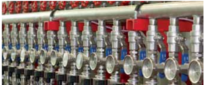
Cooling water distribution station.
