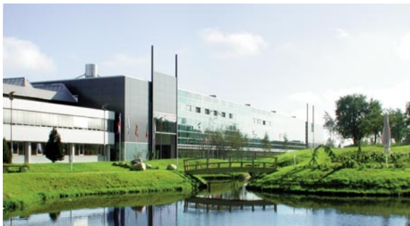
Assembly Halls with Development and Test Centre
