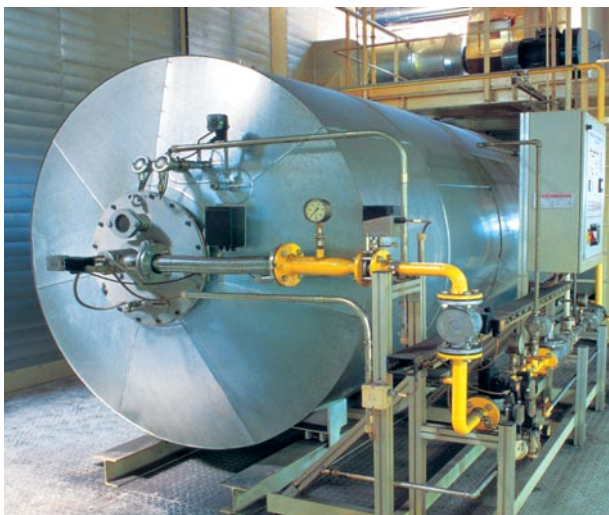
Exhaust air purification with thermal oxidation
