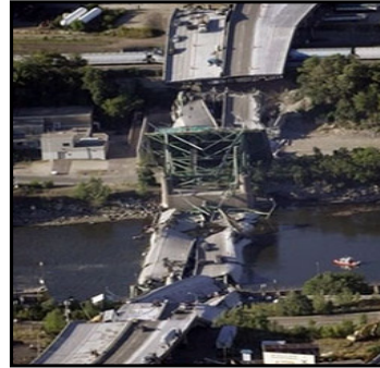
Figure 2 I-35 BRIDGE COLLAPSE: MINNEAPOLIS, MN (AUGUST 2007)
