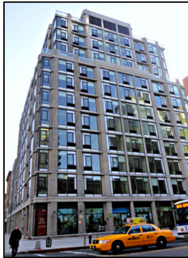
LUMIRA ® AEROGEL USED TO INSULATE WINDOW GLASS ON NYC APARTMENT BUILDING
