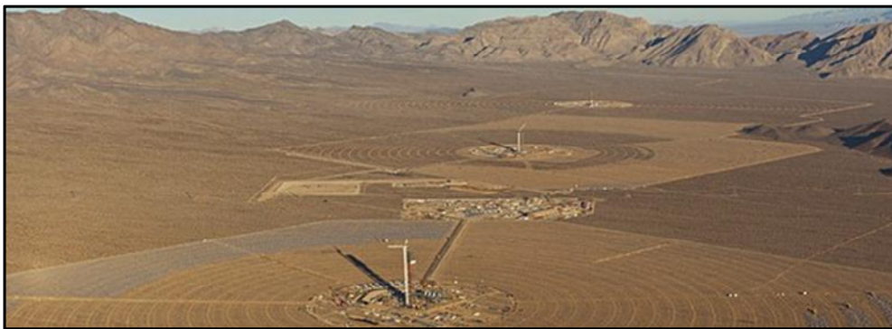
CONSTRUCTION OF THE ISEGS
