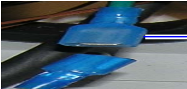
Figure 23. Cable connection between shippable sign sections.
