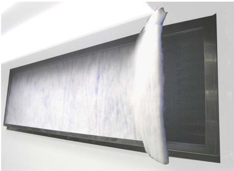
4. If the air vent filter needs cleaning, wash it using warm water and dish cleaning liquid. Rinse the filter in clean water. Then dry the filter with a clean cloth.
