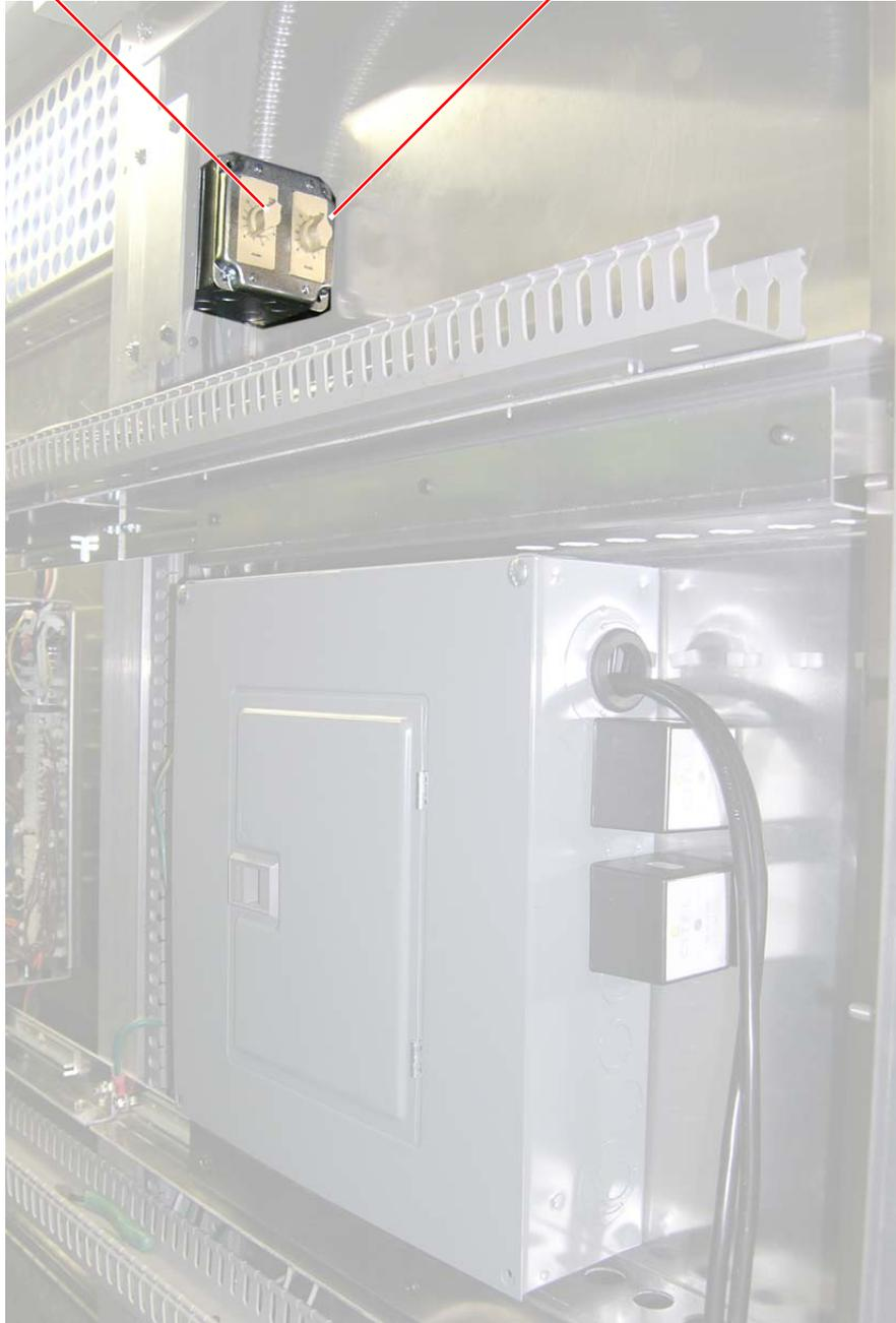
Figure 1: Lighting and fan timer switches
