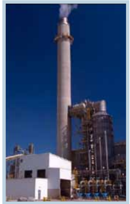
300' chimney with C-276 steel liner to service a wet scrubber stack on a cement plant in Texas
