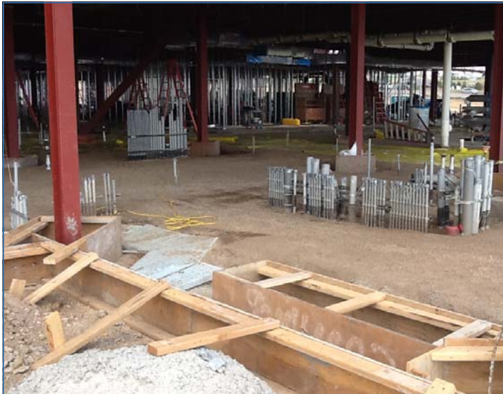
A look into the future interior of the new Veterans Affairs Clinic, currently under construction.
