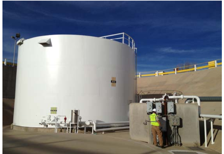
Pictured is the fuel station project at Peterson Air Force Base.
