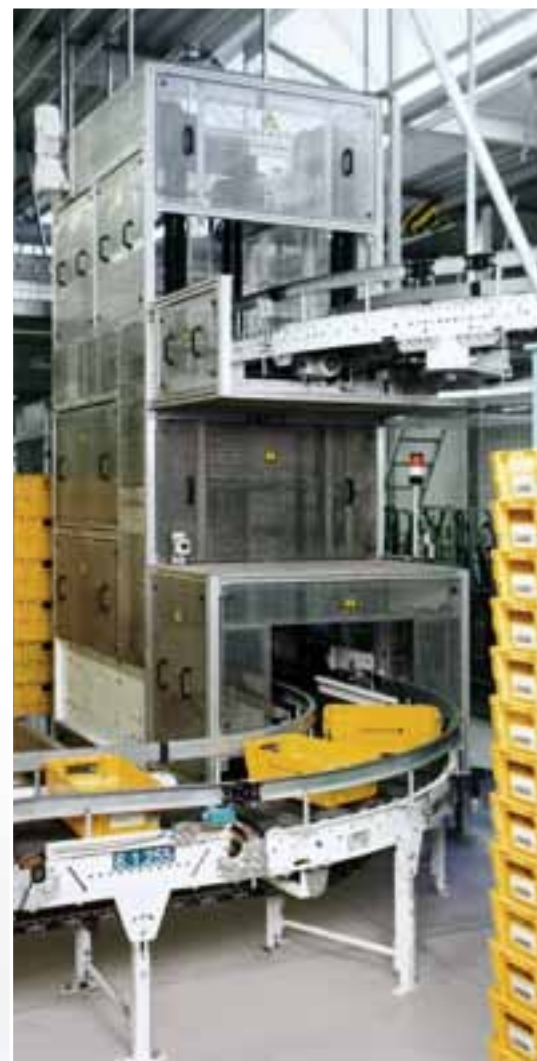
C-conveyor in mail distribution centre
