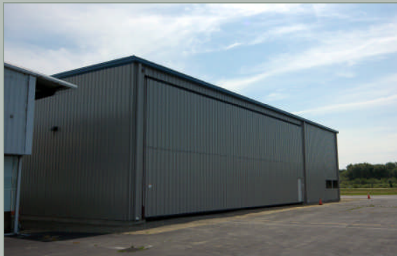
Hangar space now available. 70 foot door.
