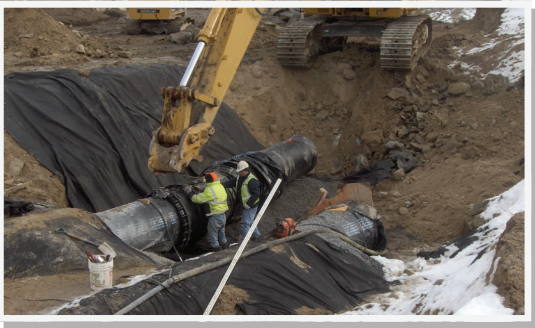
Runway Safety Area and waterline construction at the Runway 23 end - Photo courtesy of Airport Solutions Group sub-consultant Keville Enterprises, Inc.
