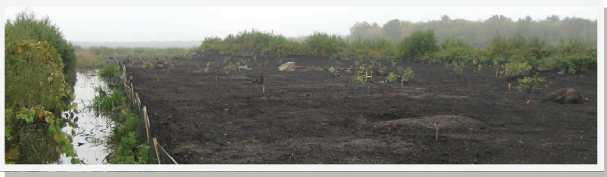
Mitigation construction for Eastern Box Turtle habitat - Photo courtesy of Airport Solutions Group sub-consultant Keville Enterprises, Inc.
