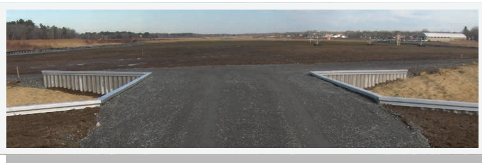
RSA construction at the Runway 5 end - Photo courtesy of Airport Solutions Group sub-consultant Keville Enterprises, Inc.
