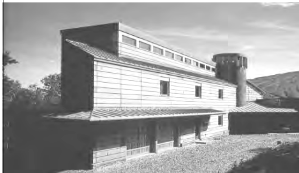
Carwill House Vermont William Pederson
