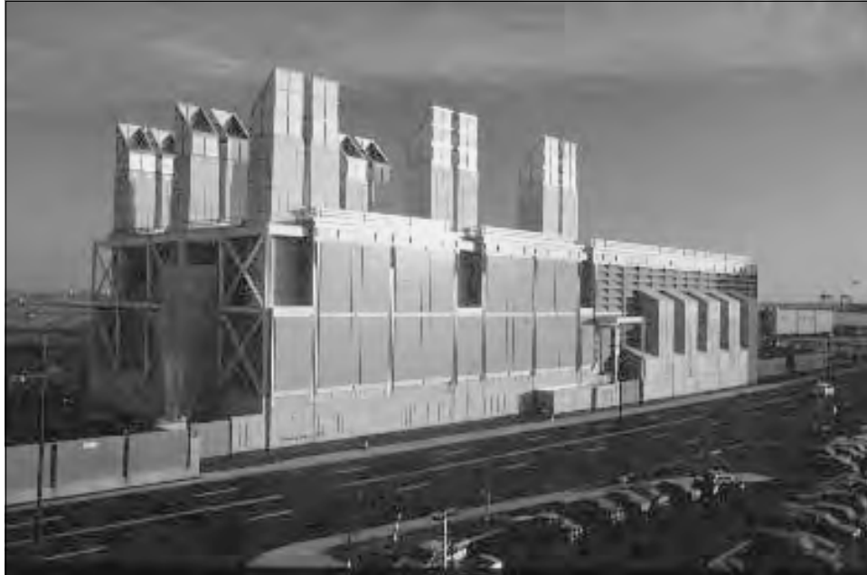
Central Artery/Tunnel Project - Ventilation Building No. 7 by TAMS/Wallace/Floyd Associates/Stull Associates
