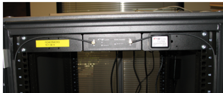
Figure 12 R150 Rack Temperature Tag shown as Reader Bracket Mount
