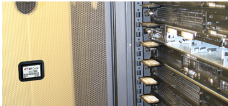
Figure 12 R150 Rack Temperature Tag shown as Reader Bracket Mount
