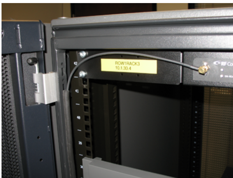
Figure 2 Antenna Mounted in Rack
