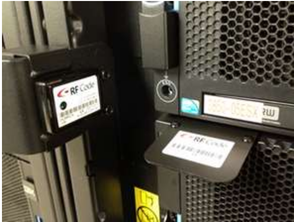
Figure: An R155 temperature-humidity sensor mounted on the inside of a rack (left side of photo) near an R104-I IT Asset Tag (right side of photo)
