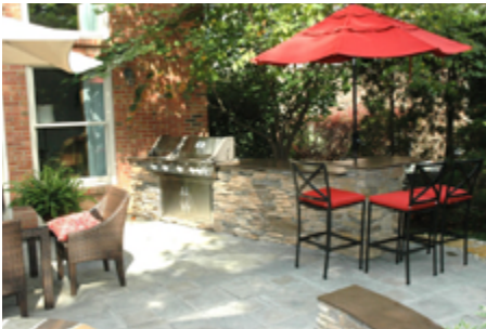
A combination grill was set into a retaining wall that surrounds this patio. There is a counter with an overhang for setting down dishes and a section that forms a bar.
