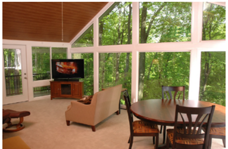
A traditional three-season room usually requires two feet of walls in the corners for wind bracing. This homeowner wanted as much glass as possible to bring light into a home surrounded by tall trees. A custom designed and engineered sunroom provided the best solution. The windows use Low-E glass with special coatings that reflect heat back inside to warm the room in the winter and reflect solar energy away in the summer, all while minimizing damaging UV rays which cause furnishings to fade. The room is elevated and opens onto a deck.
