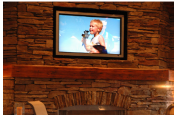
This television designed for outdoor use is protected in this open sided gazebo. The exterior is designed to resist moisture, cold temperatures, snow or salt air. The fireplace is a Lennox ventless gas fireplace. Walls are southern ledgerstone.
