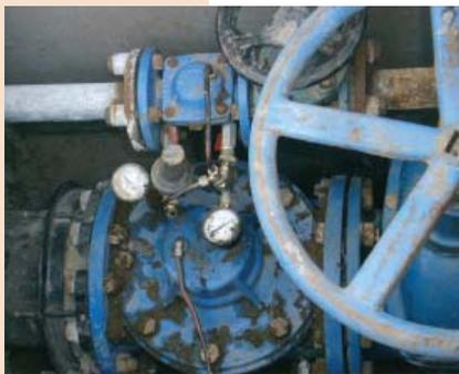
Soujah replaced the faulty pilot with a Singer Model 160 Pressure Reducing Pilot. Immediately, the valve began to regulate the pressure. Needless to say, Rahman and his team were relieved and pleased.
