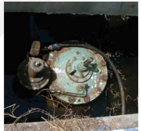
“The altitude pilot is a three-way pilot operated by a spring and diaphragm,” says Eugene Bahia, a Singer Valve instrumentation specialist. “The pilot precisely controls the water level in a reservoir because it accurately senses the hydrostatic head.”
