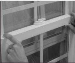
Depress the tilt latches located on the top of the sash. (one per side, push toward the center/lock)
