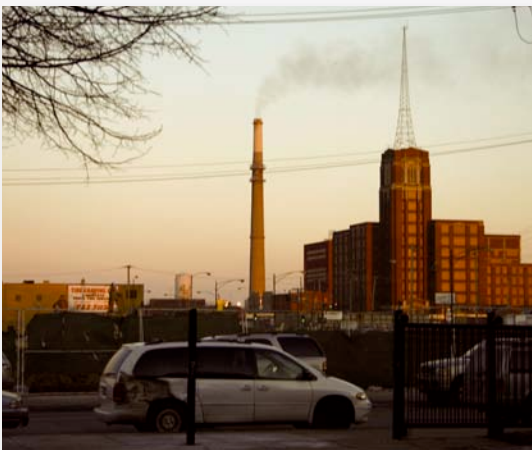
Coal-Fired Power Plant, Chicago
