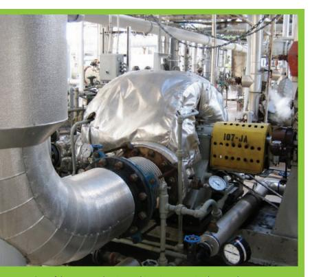
One of the new condensing turbines in ammonia plant #2; these new turbines are reducing energy use by 228,000 MMBtu annually.
