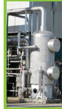
A loop dehydrator installed in ammonia plant #2 is also saving the plant 228,000 MMBtu per year.
