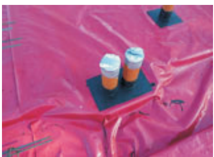
Install Radon Barrier
