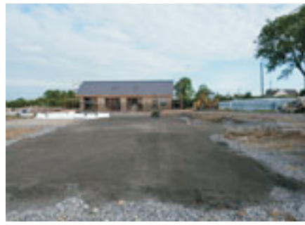
Limestone binding used to level off
