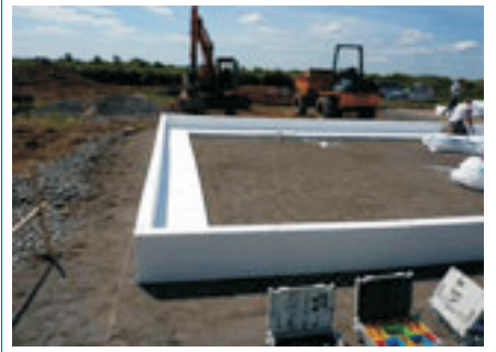
Install 1st layer of Ringbeam element
