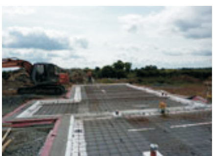
Install steel mesh & UF Heating Pipes
