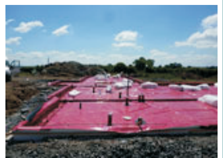
Ensure full Radon Coverage
