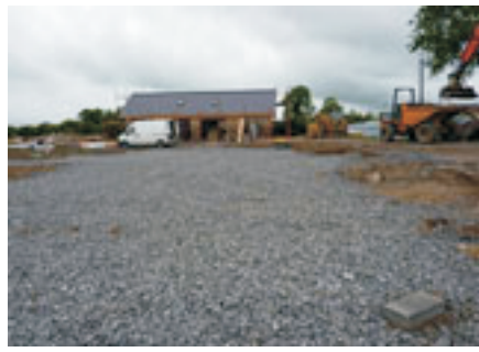
Compress 18-35mm Stone in Layers
