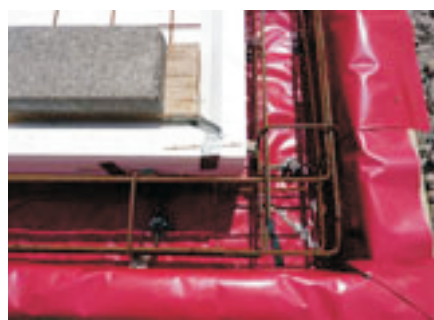
Install Steel in Ringbeam
