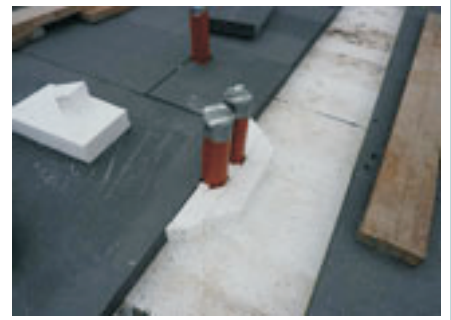
Insulate around pipes
