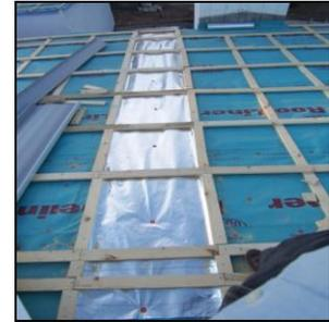
Four temperature and relative humidity sensors were installed on top of the foam insulation below the roof decking in each of the bays. The data logger recorded temperature and relative humidity data at 15 minute intervals.
