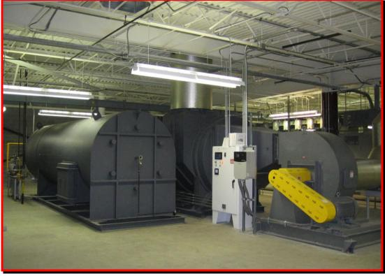
The worlds largest automotive manufacturer recently installed our QUADRANT SR-Series Thermal Oxidizer for use at destroying CO and VOC emissions from their engine test cell facility. The test facility houses several engine, transmission, and chassis dynamometer's. The manufacturer demanded a system that would provide the highest uptime reliability and highest performance.
