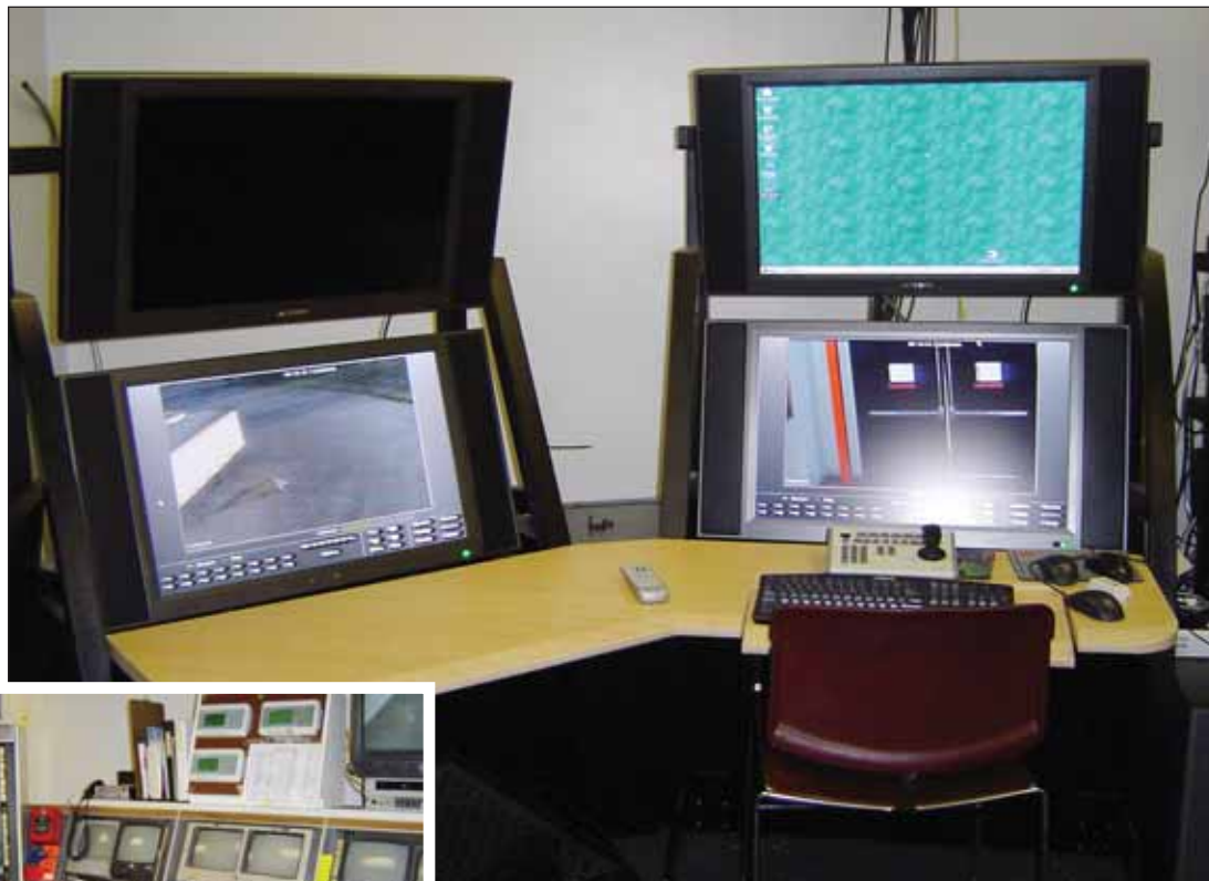
Left: An old security console with outdated equipment was replaced by Security 101, Marietta, Ga., with a new console shown here under construction (above). It features four 32-inch LCD flat-screen monitors and integrates access control with CCTV and intrusion devices.
