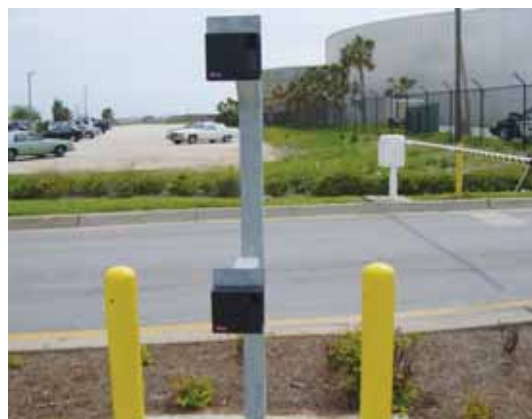
An ID card reader for vehicle traffic also was installed by Anteon at a U.S. port.
