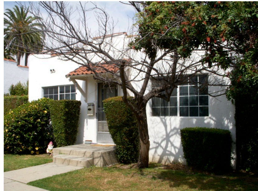
One of the existing bungalows at 1408-10 Rock Glen Ave
