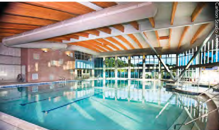
▲ A V-shaped pair of 10-in.-diameter HSS columns support a 94-ft-long girder, springing from the center of the pool from a common base plate.
