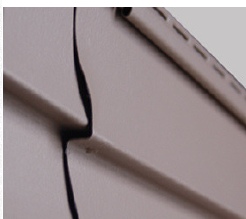
EXAMPLE: Overlapping vinyl siding seams may leave an undesired look.
