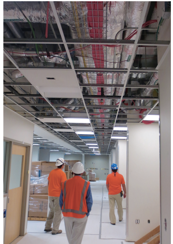
Left-to-right: Lance Lines, CIS on-site project manager; Larry Smith, manager of data cabling with Mercy; and Eddie Ouellette, CIS site manager, inspect pathways within Mercy Hospital Joplin's intensive care unit.
