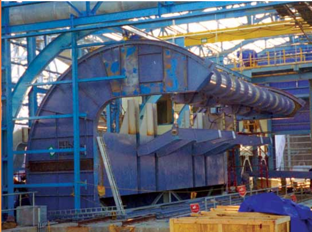
Wagon Tippler under construction
