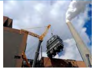
Installation of Fluid Bed Dryer for Lignite
