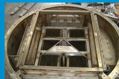
Retrofitting of Existing Tank
