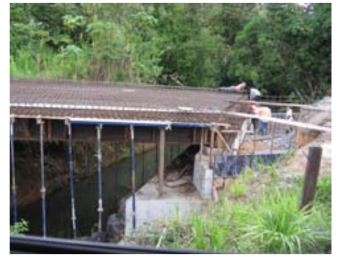
New bridge nearly complete in San Buenas
