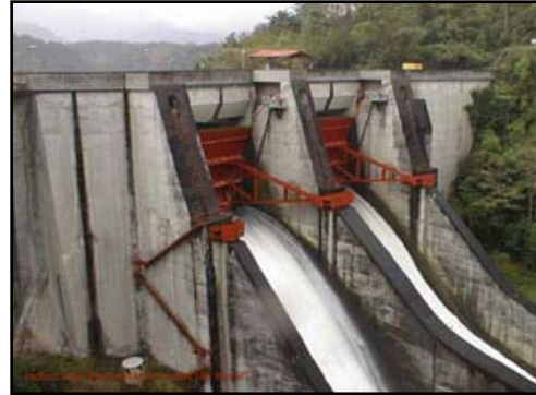
Cachi Hydro Station
