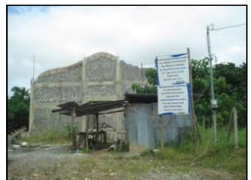
New church under construction in Ojochal
