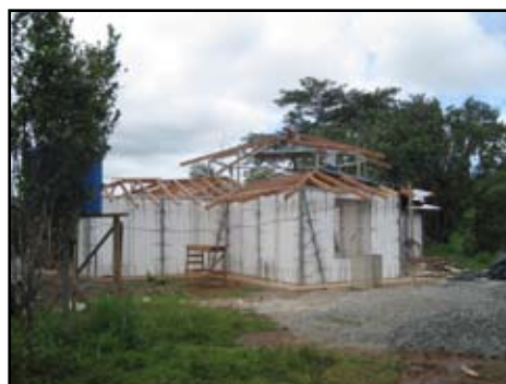
New guest house going up
