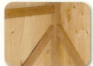
Oak Post & Beam-Style Framing
