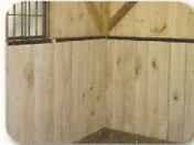
4' High Oak Kickboard with Steel Chew Guard (Standard on Stall Barns)
