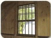
Powder-Coated Steel Grill Over Windows (Standard on Stall Barns)
