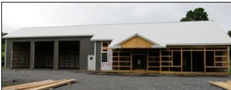
MAVES building during construction in June ...
