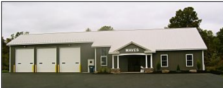
... and nearing completion in September
