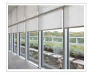
Installing one shade drive to operate multiple fabric panels creates a cost-effective solution without sacrificing automation or daylight harvesting.
