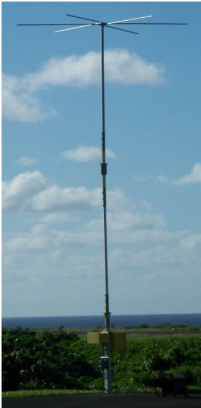
SAC 34 ft. Land Mast Antenna in Samoa
