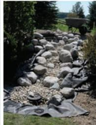
Place rockwork at the end of the stream area. Complete the waterfall & stream area. Be sure that the Cascade box remains level throughout the process so that the water flows out evenly when finished.
