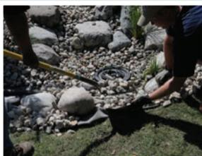
in the area around the Cascade box making sure not to place any rockwork that will pull away the liner from the Cascade box. Begin filling the basin with water while completing the rest of the steps. Wash off any dust from your rockwork.
