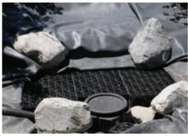
Install the waterfall and stream liner (if separate from basin liner). Lay the liner so that there's enough to overlap the basin liner by at least 6" and also so there's enough liner at the top of the waterfalls to attach to the Cascade Box.
