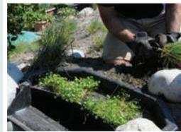
Build up the area behind the Cascade box using rockwork and soil or gradually slope the soil back to grade. Finish all
