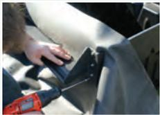
Attach the liner to the Waterfall Box. Refer to the instructions provided with the waterfall box for assistance. Once the liner has been installed on the waterfall box you can complete rocking in your waterfall and streambed.
