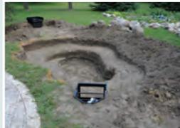
Excavate pond with at least two levels. Excavate the pond to depth of first level. Spray out the area that will become the deeper portion of the pond. The use of a laser level is very helpful in determining whether the sides of your pond are level all around but a string level works too. Dig at 90° angles.
