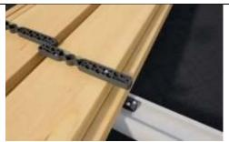
Step Five: Now line up your next rows of deck boards and start fastening the Deck Gliders to the bottom of each deck board. Alternate the spacing left and right for each row of deck boards so they will fit into the Aluminum System Profile joist properly.
