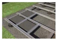
7.) Double-check your completed frame and make sure everything is squared up and level before installing your decking boards.
