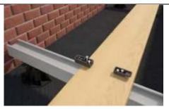
**Step Three**: Screw the male end of the Glider Starter Clip into the bottom of the deck board and the "cut off" end of the Deck Glider on the other edge of your deck board. (Pre-drilling pilot holes is required.)
