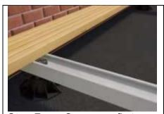
Step Four: Once your first deck board is lined up and in place, fasten your first deck board by screwing the exposed edge of the Deck Glider to the Aluminum System Profile into the two screw holes.
