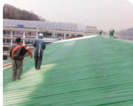
Gymnasium Roof Foam Protection
