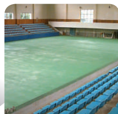
Floor for multipurpose stadium
