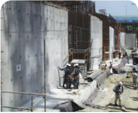
Waterproofing of underground structure in Incheon International Airport
