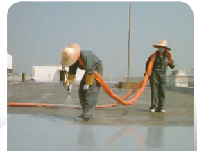
Wastewater Treatment Facility Roof Waterproof
