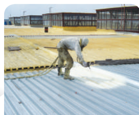
Roof Insulation of Warehouse
