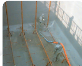
Chemical Wastewater Treatment Facility Waterproof
