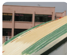
Roof Insulation of Gymnasium
