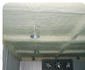
Inside Insulation of Cold storage house
