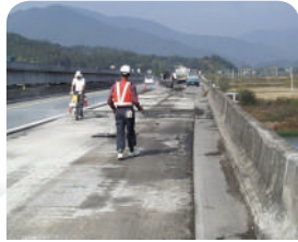
Bridge deck waterproof
