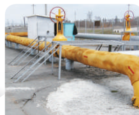
Water pipe Insulation for heating steam
