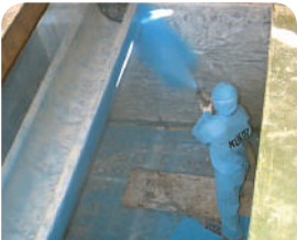
Tab Water Treatment Facility Waterproof
