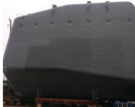
Fire resistance for LPG/LNG cargo protection
