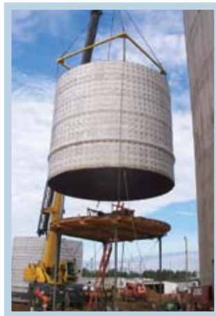
Right: 531' tall completed chimney shell at AEP Welsh Generating Station, TX Left: Steel liner installation
